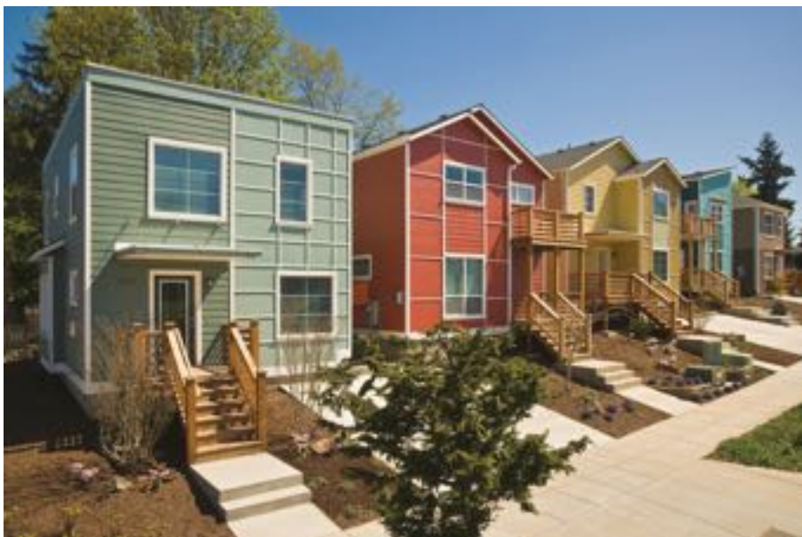
Green and affordable housing in Portland. ecobuildingpulse.com
